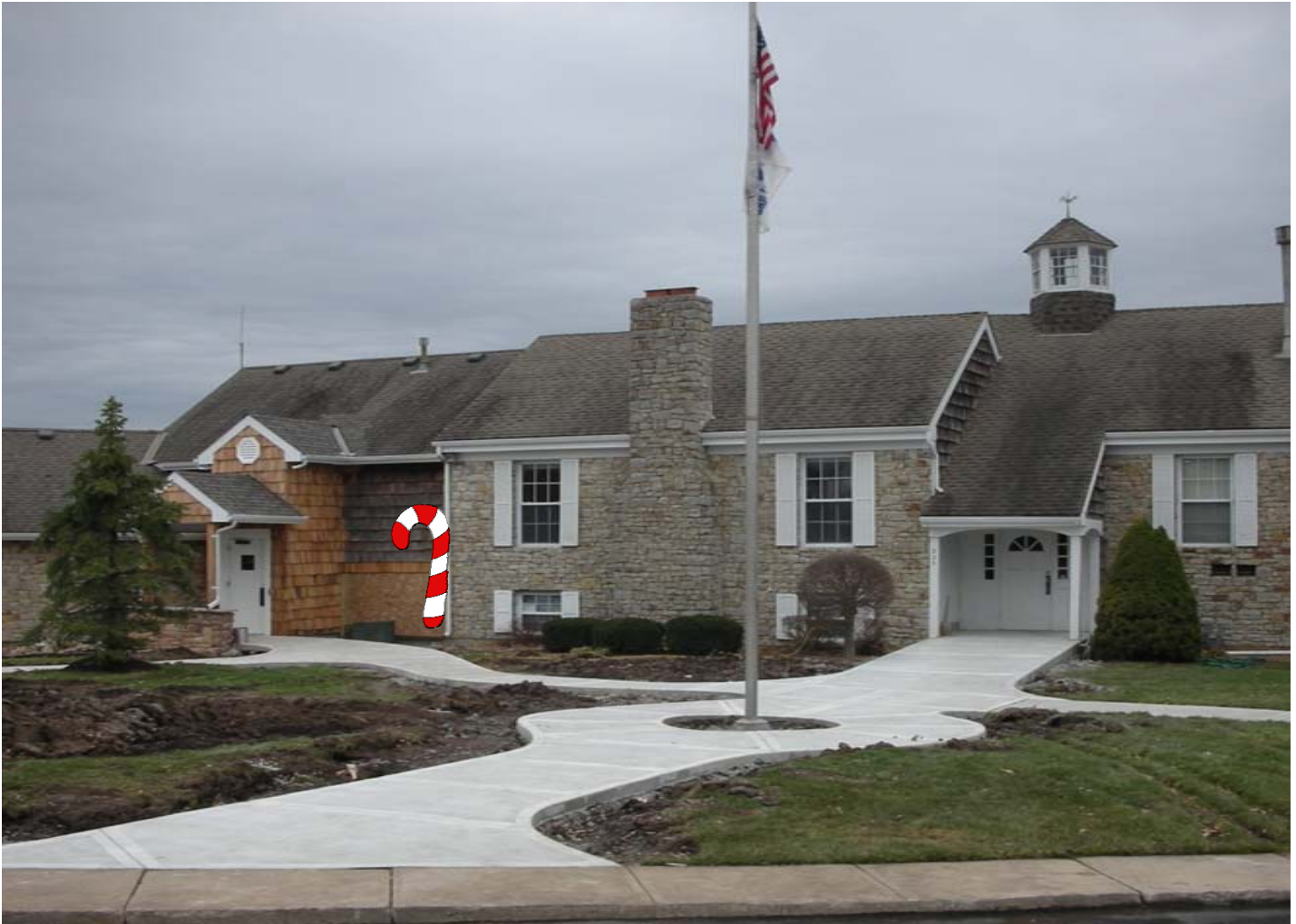
Clubhouse Interior/Exterior Transformation, Cost: $200,000
