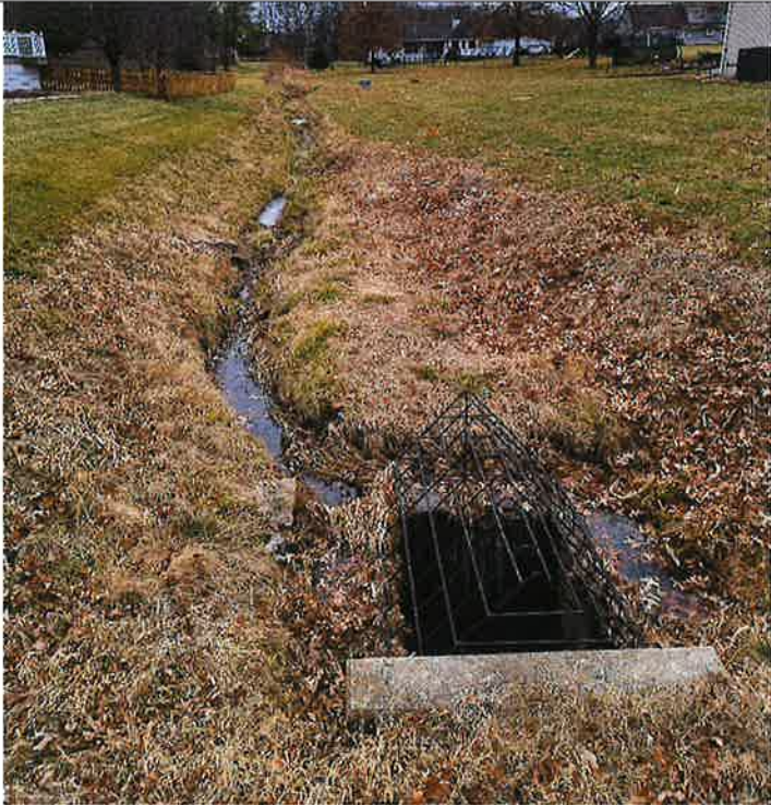
View of upstream channel, culvert inlet, drop structure, debris catcher (December 2022)
