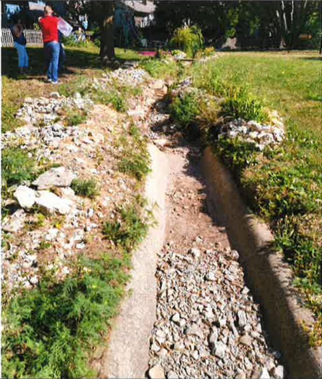
At downstream flume, looking upstream at channel
