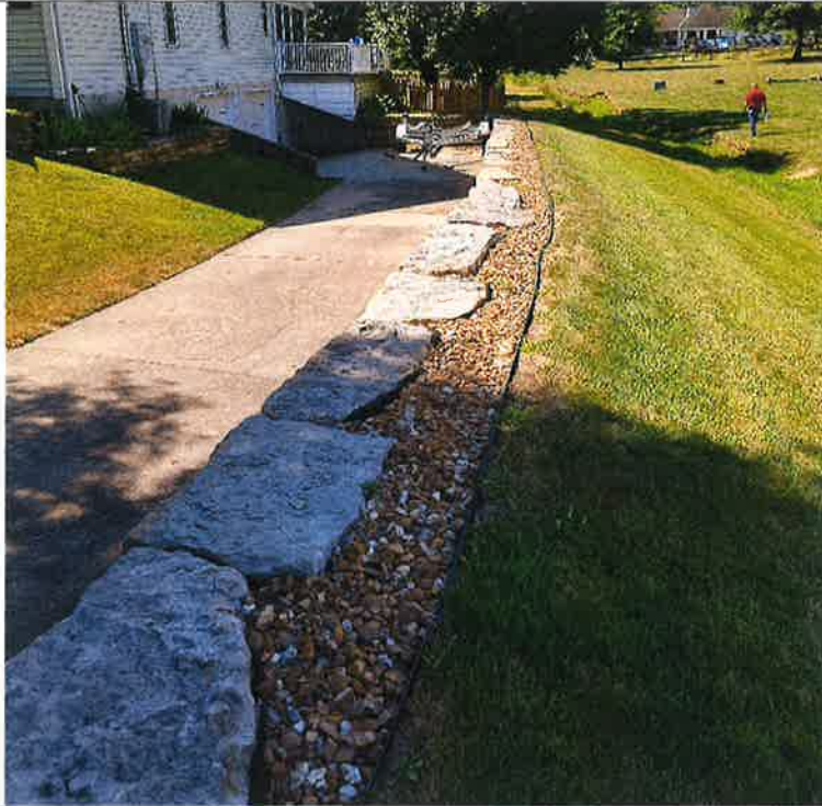
Retaining wall at 5271 SW Raintree Pkwy residence, upstream channel at right
