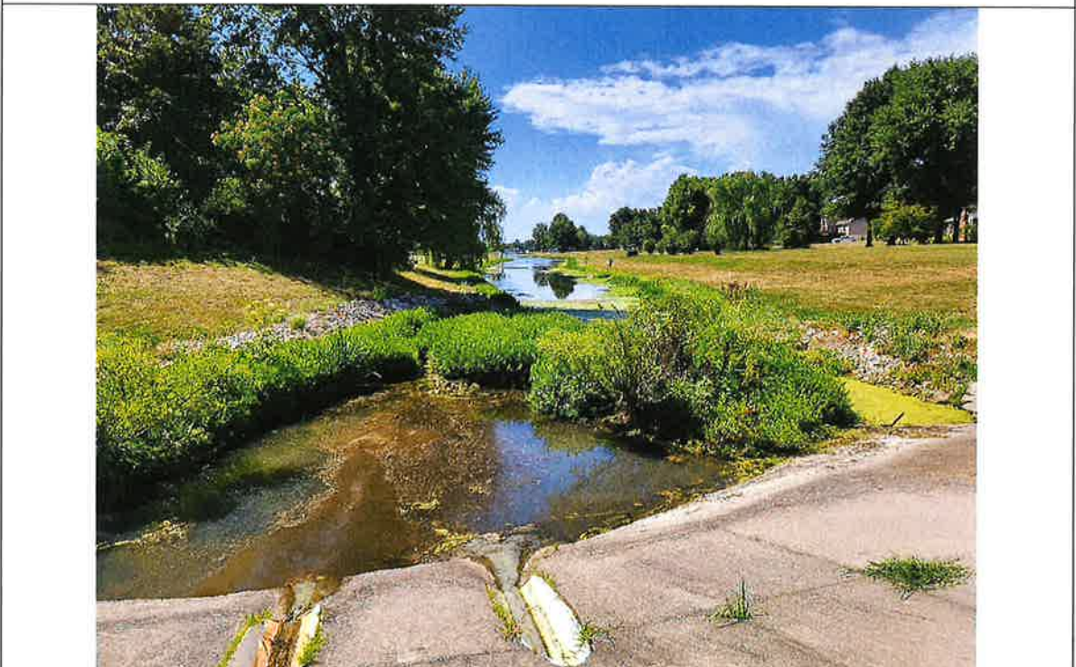
Standing on detention pond overflow structure looking downstream at lake
