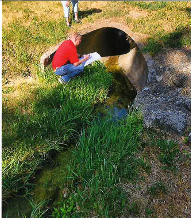
Inlet end of culvert under SW Hidden Cove Dr
