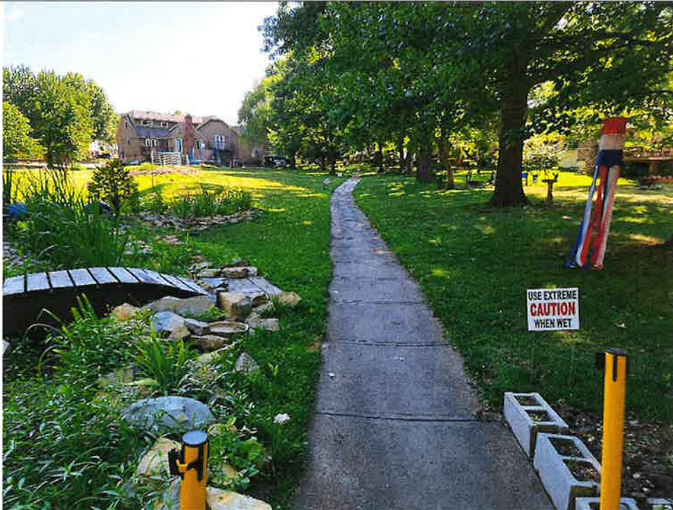
Downstream end of concrete flume between Pendant/Royale backyards, looking upstream
