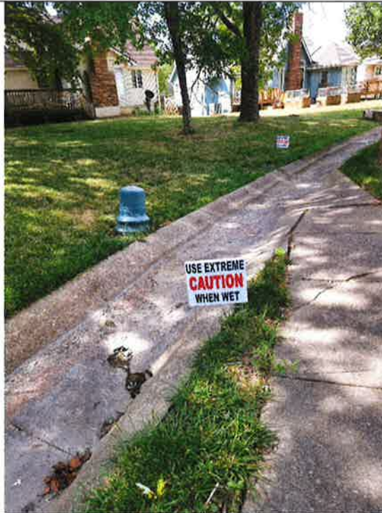
Sidewalk and flume between Pendant/Royale backyards at upstream end, looking downstream
