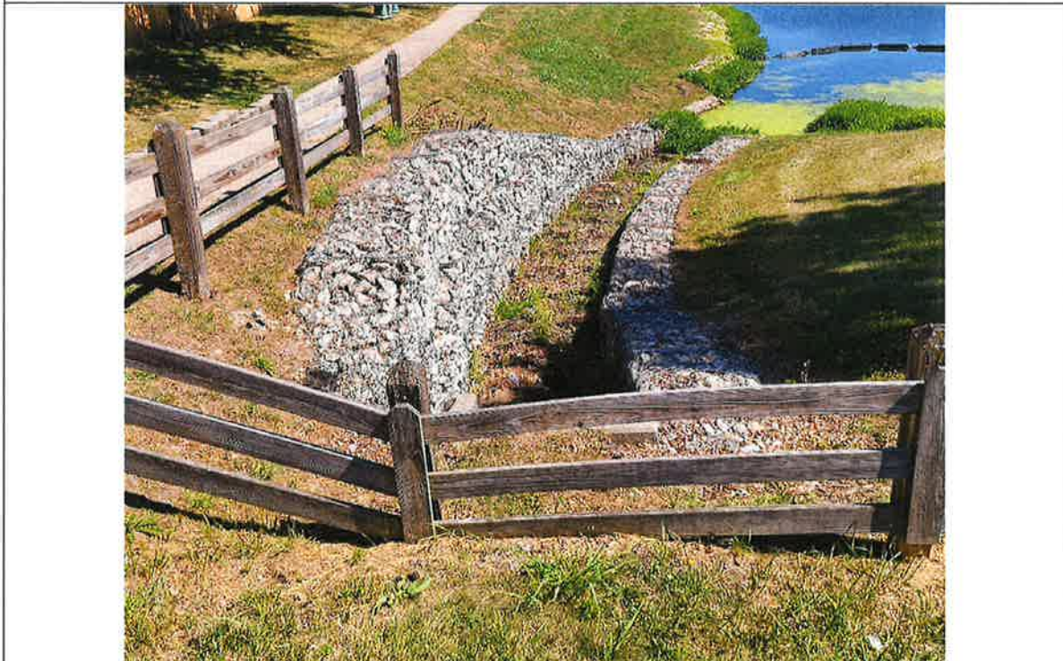
Gabion baskets lining channel banks downstream of culvert outlet
