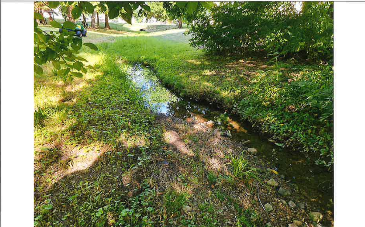
Looking downstream at channel from end of concrete flume
