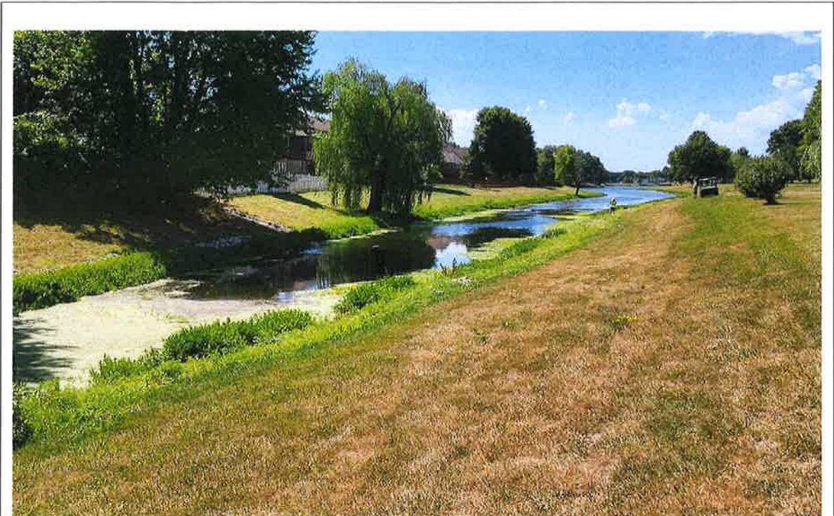
Standing at upstream end of Sunset Cove, looking downstream
