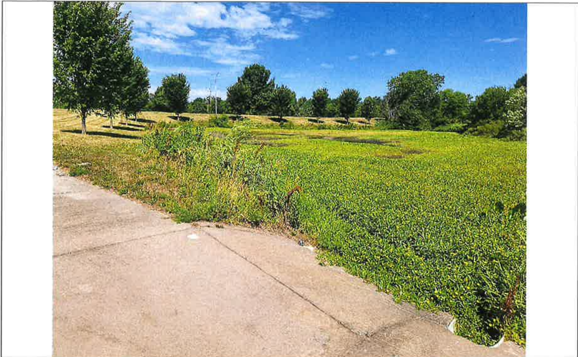
Standing on detention pond overflow structure looking upstream at pond
