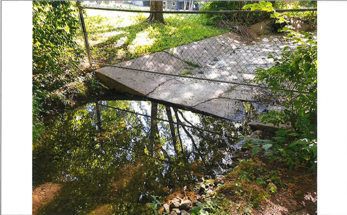
Downstream end of concrete flume, looking upstream
