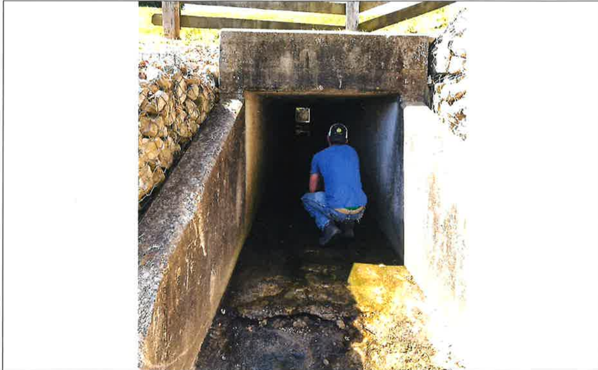
Culvert outlet, looking upstream
