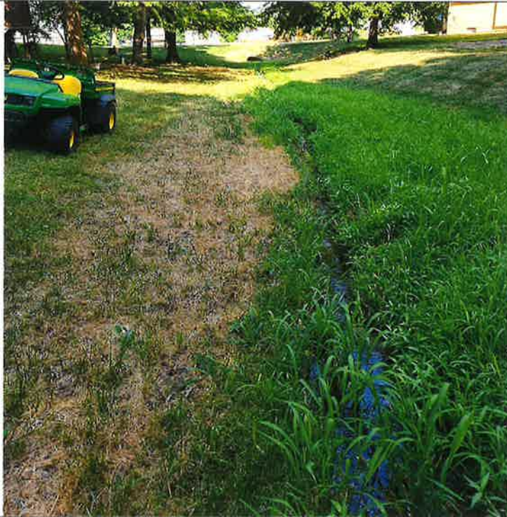
Channel, looking downstream at culvert under SW Hidden Cove Dr
