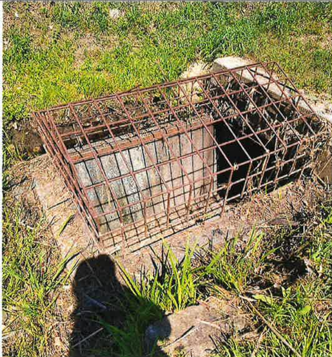
Culvert inlet, drop structure, debris catcher (July 2022)
